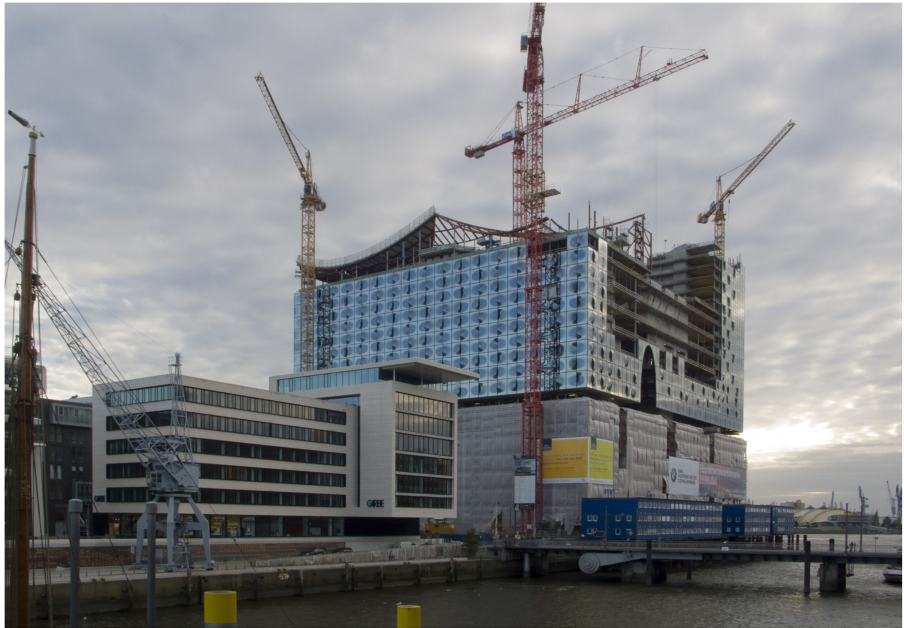
Figure 4. The Elbphilharmonie, Hamburg, Germany, under construction, 15th September 2010 (Photo: Gunnar Klack, CC BY-SA 4.0)
