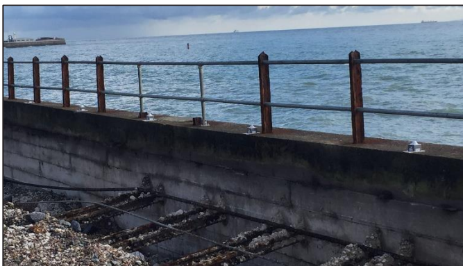
Figure 2.1 Installed sensors on top of Dover Sea Wall
