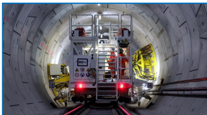
Figure 18: Automated tunnel drilling machine working in its operating configuration
