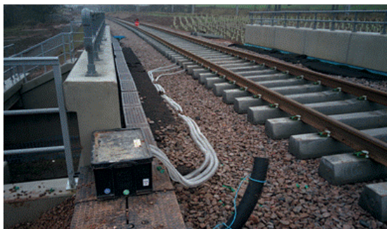
c) Self-sensing sleepers on bridge
