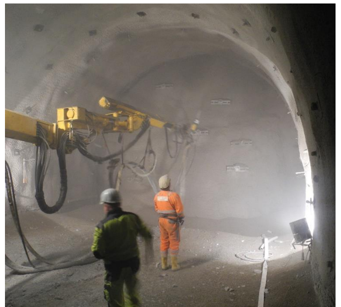
Figure 5 Spraying of the second layer of shotcrete of the top heading
