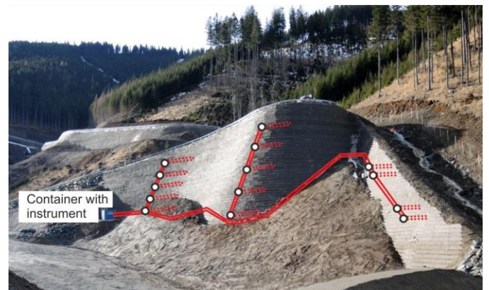
Figure 14 Fibre optic measurement loop at the reinforced earth structure in the Longsgraben valley
