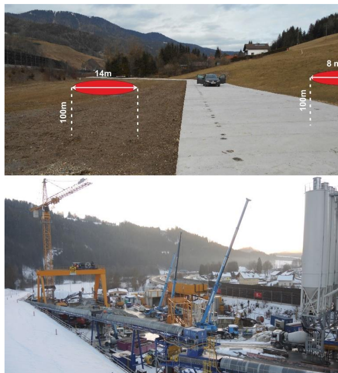
Figure 19 Construction site after installation of the fibre optic sensing cables in 2016 (top) and in winter 2018 (bottom)
