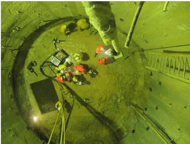
Figure 9 Vertical view down the shaft during construction at Göstritz
