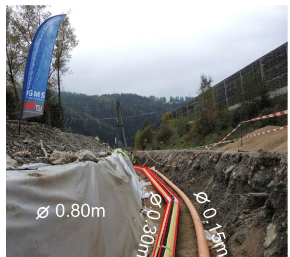
Figure 17 Relocation of the pipelines at the Grautschenhof construction site
