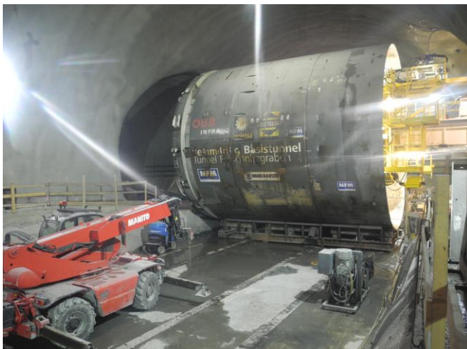
Figure 21 Drilling head of the tunnel boring machine in the starting cavern at Fröschnitzgraben
