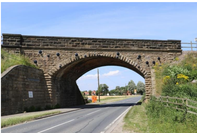
Figure 1 Bridge CFM-5, as viewed from the south
