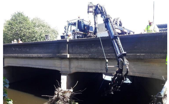
Figure 3: BridgeCat vehicle taking sonar scans before repair
