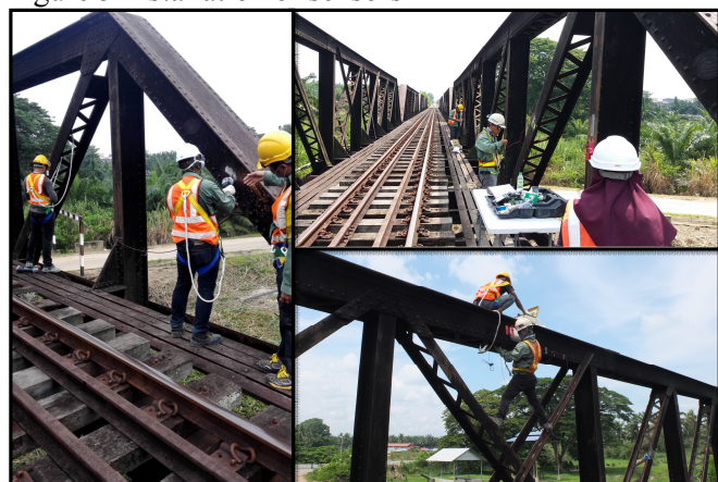
Figure 5 Installation of sensors
