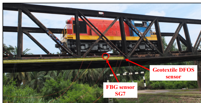
Figure 5 Installation of sensors
