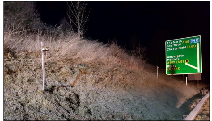
Figure 4.3 Triaxial tilt sensors attached to stakes driven into the earthwork beside the A38 road, Ripley.
