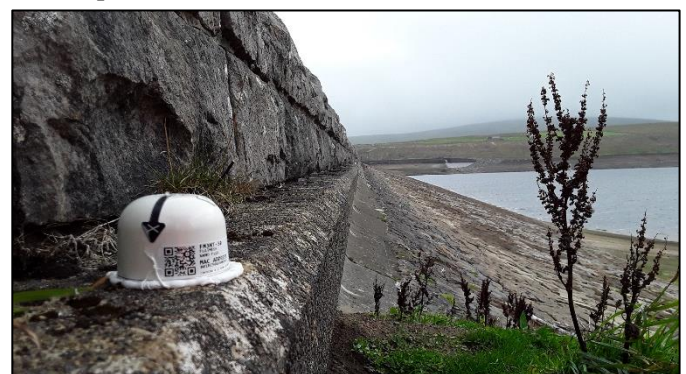
Figure 4.4 Nano+ triaxial tilt sensor installed on Burnhope Reservoir's wave return wall.
