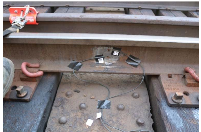
Figure 4 Strain gauges on the rail over top of floor beam
