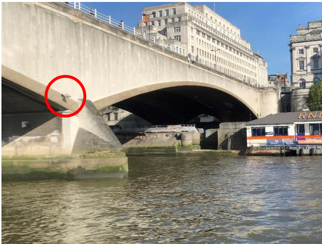
Figure 5 Aluminium corner reflector (circled) installed on bridge pier alongside ATS prism targets.
