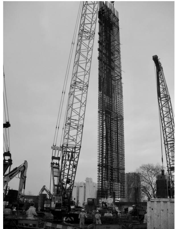
Figure 4 Installation of instrumented reinforcement cage
