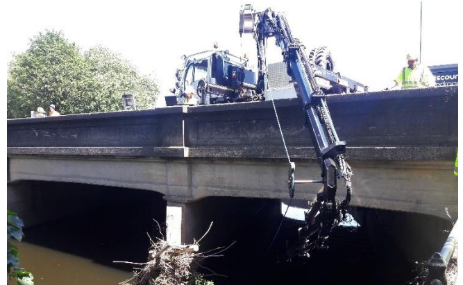
Figure 3: BridgeCat vehicle taking sonar scans before repair
