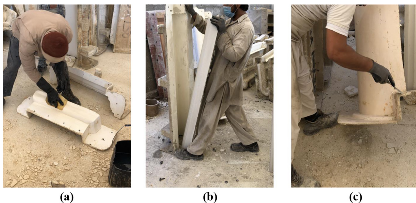
Figure 2. Workers performing mold oiling, mold opening and mold cleaning tasks
