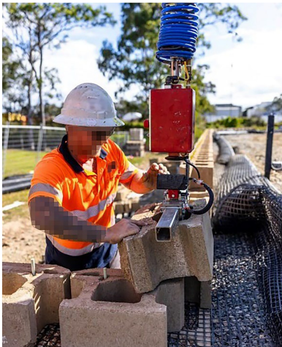
Plate 2. A close-up view of the bricklayer positioning the CMU in place as the MULE suspended gripper and controller hold it
