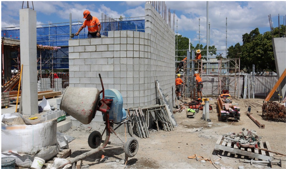
Plate 3. Challenges setting up the MULE on unstructured sites mean bricklayers still manually lay CMUs at height without its assistance
