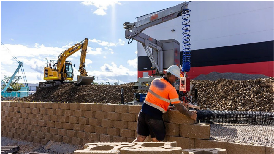
Plate 1. A bricklayer guides a CMU into position using the MULE system. The MULE’s arm pivots as the bricklayer aligns the CMU on the retaining wall Source: Armstrong Bricklaying. Used with permission
