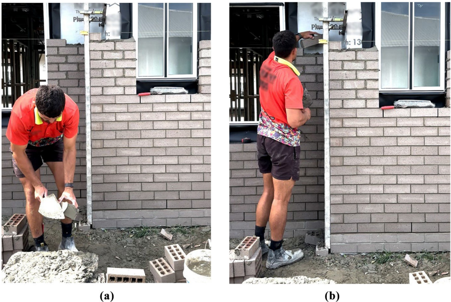
Plate 5. Site photographs showing manual bricklaying tasks. (a) A bricklayer bends down to apply mortar (“mud”) evenly across the brick face. (b) Brick placement in a constrained area requires stretching and navigation around corners, string lines and structural features (2025). Images used with permission in accordance with ethics approval (Approval Number: 8581)
