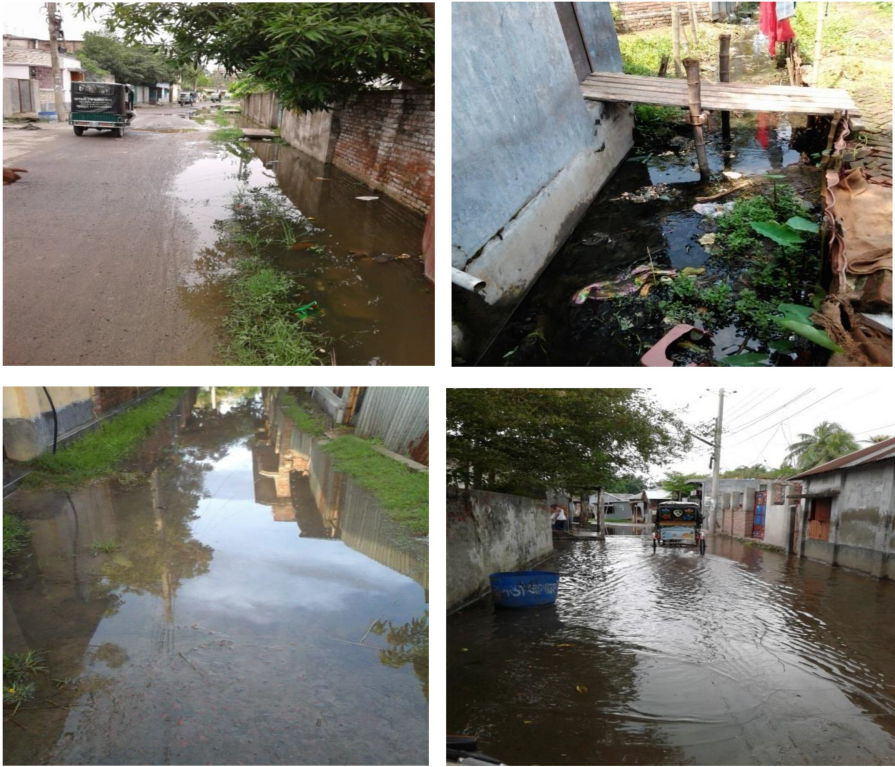
Plate 1. Visual of existing waterlogging problem
