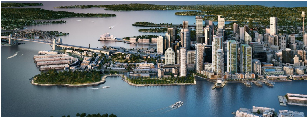
Figure 5. Barangaroo in Sydney is Australia's largest urban regeneration project (image: courtesy of Lendlease).
