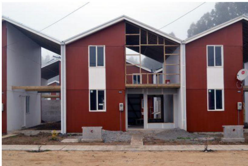
Figure 1. Housing by Elemental in Constitución, Chile. Individual two-storey half houses for informal, incremental self-building by the residents (2010). Aravena has championed an approach he describes as 'incremental', in which governments fund construction of 'half a good house', with residents completing the other self-built portion informally as resources allow (photo courtesy of Elemental).
