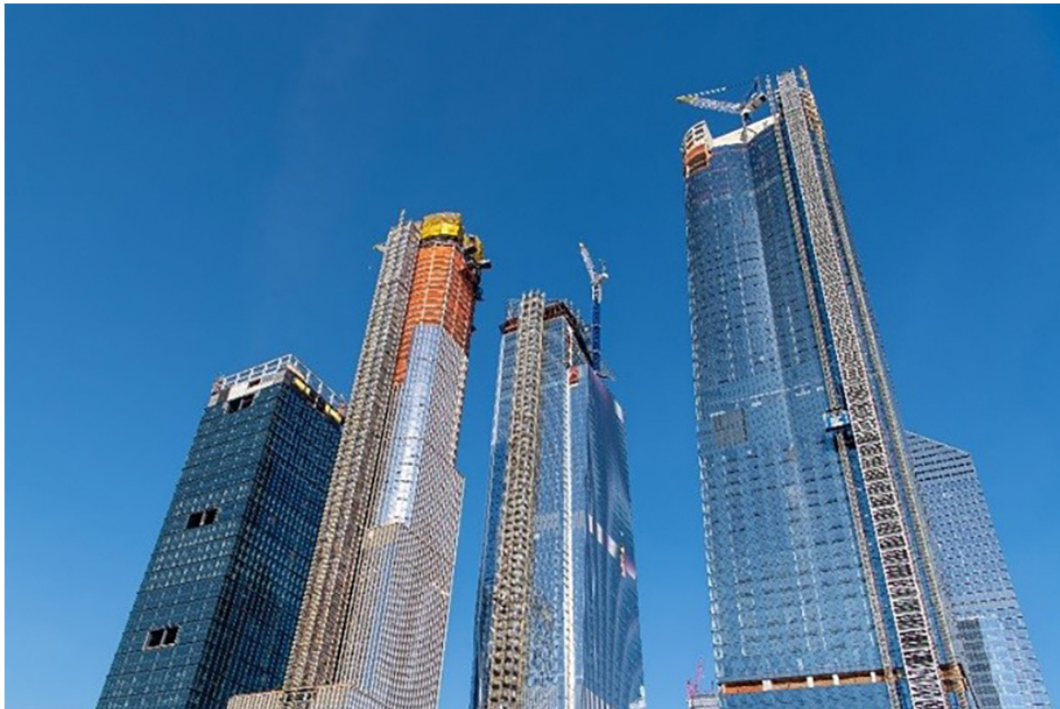
Figure 4. Construction of office and residential towers at Hudson Yards. Source: © Jim Ekstrand / Alamy Stock Photo.
