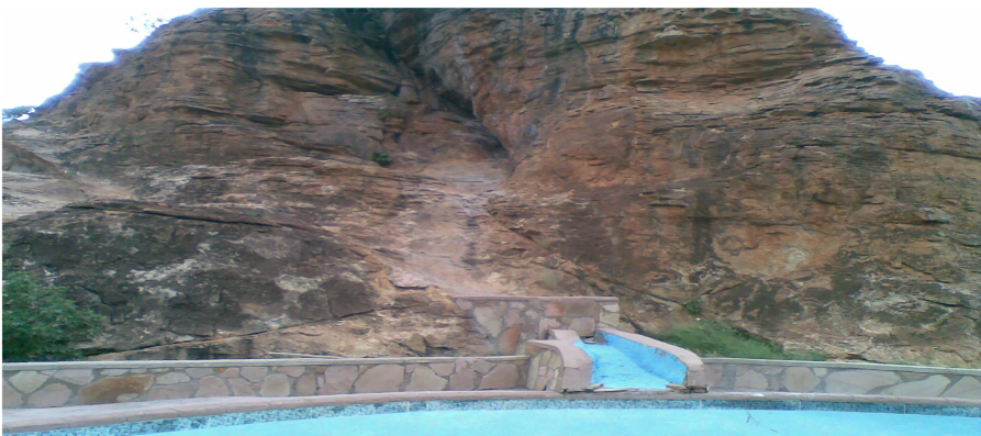
Plate 2. Swimming pool is attached to the mountain hill as a source of water in a private lodge entity next to the big tree nature reserve. Source: Author, 2019
