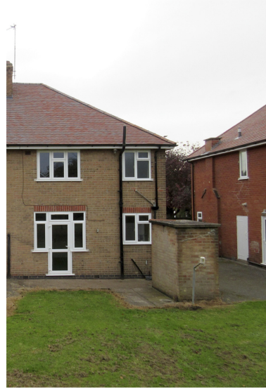
The test house from the rear (north) side (b)
