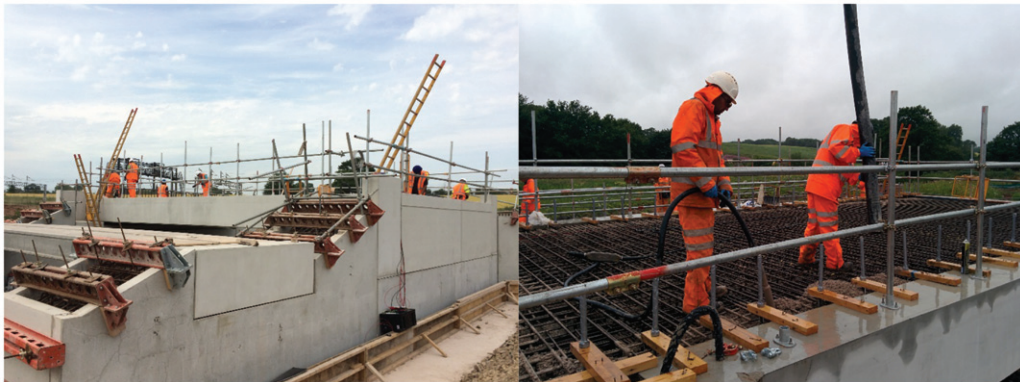
Figure 6. Bridge under construction during deck casting
