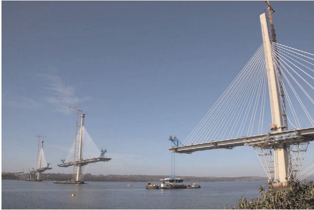
Figure 3. Cantilever method of superstructure assembly
