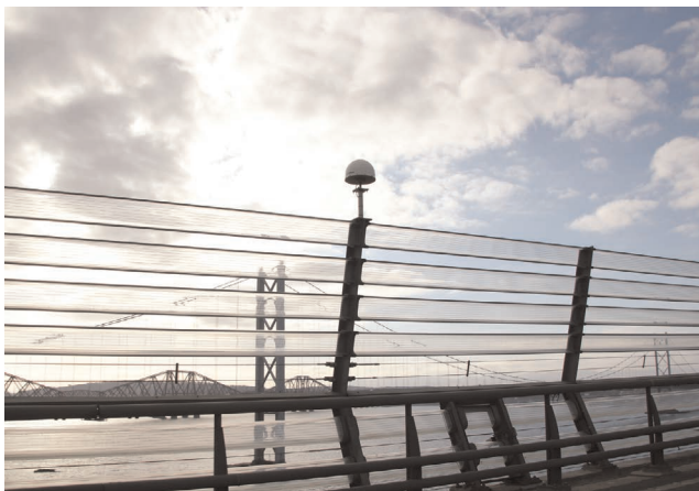
Figure 8. GNSS positioning receiver on wind shield
