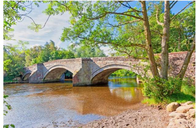
Figure 10. Pooley Bridge before collapse (Steele, 2012)
