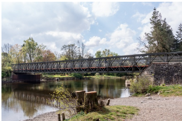
Figure 11. Completed temporary Pooley Bridge (Price, 2019)
