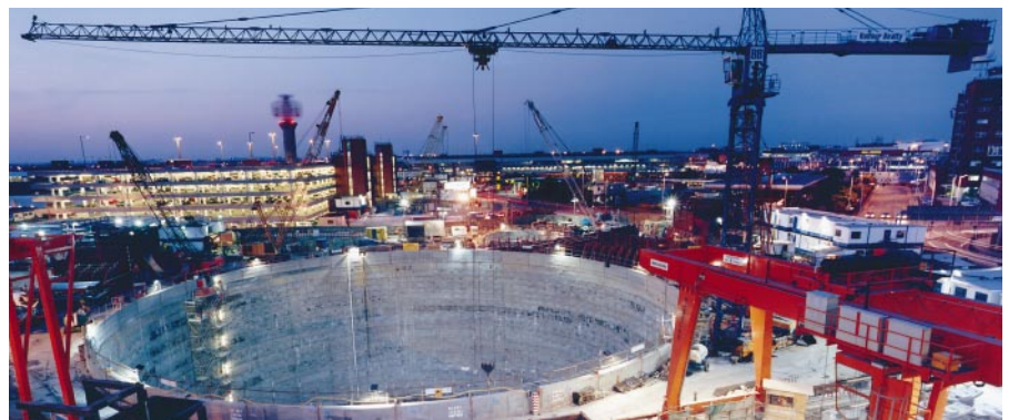
Safety lessons from the Heathrow tunnel collapse were not made available for six years
