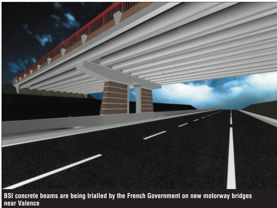
The fibre-reinforced material has a compressive strength of up to 150 MPa and tensile strength of 10 MPa
