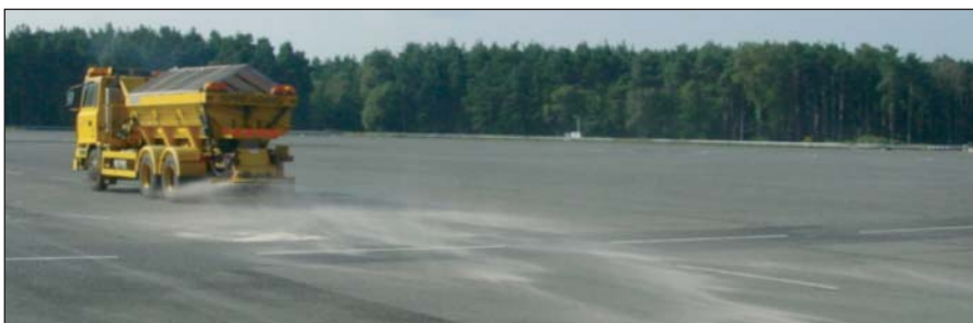
Trials at TRL Limited found that road de-icing salt pre-wetted with Safecote cut its corrosive effect by 45%
