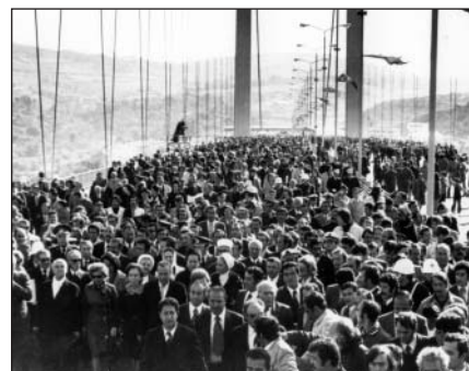
Close to disaster? Crowds on the opening of the first Bosphorus bridge in 1973 are believed to have caused an imposed loading up to three times higher than the bridge was designed for
