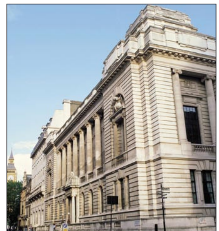
ICE's new learned society structure is designed to strengthen its position as the leading source of expert civil engineering knowledge
