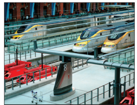
ICE plans to bring together examples of good client practice, such as the £5.8 billion High Speed 1 project completed on time and within budget in November 2007
