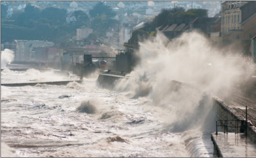
Figure 4. Resilient infrastructure – storm damage to the main railway in Devon, UK in 2014 showed how critical infrastructure is to sustaining local economies
