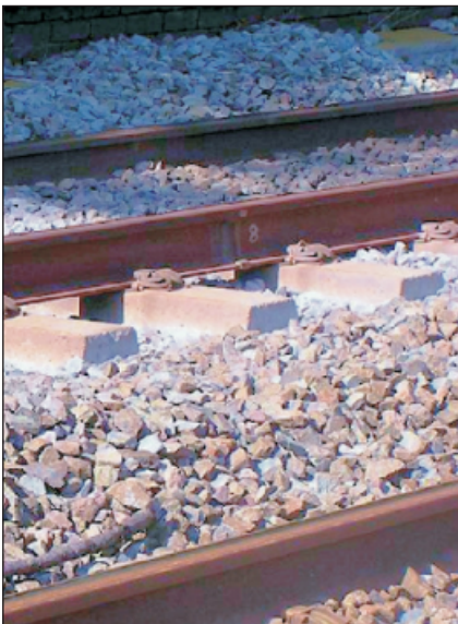
Slab track would avoid problems such as ballast migration on canted curves
