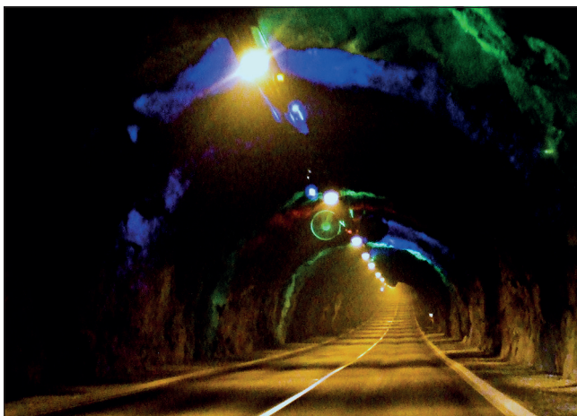
Figure 3. Norðoya tunnel was opened in 2006 (by Arne List (talk) – authors’ own work, CC BY-SA 3.0, https://commons.wikimedia.org/w/index.php?curid=4233831 )
