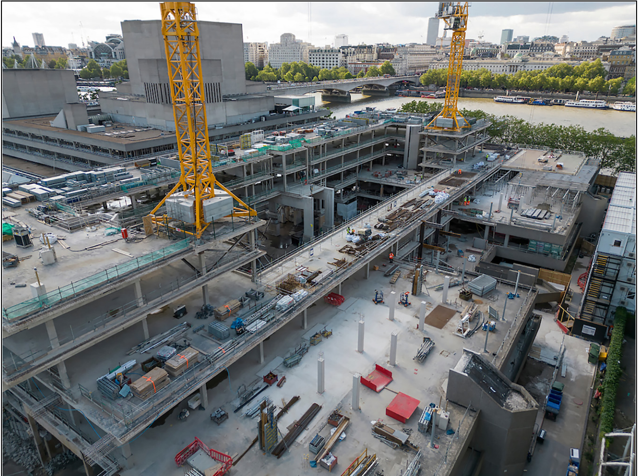
Figure 3. Demolition and construction works
