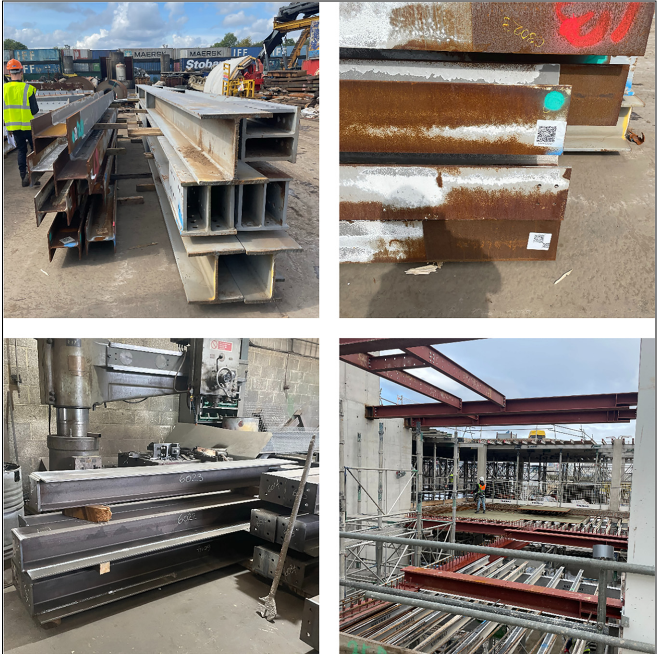
Figure 10. Reused steel process
