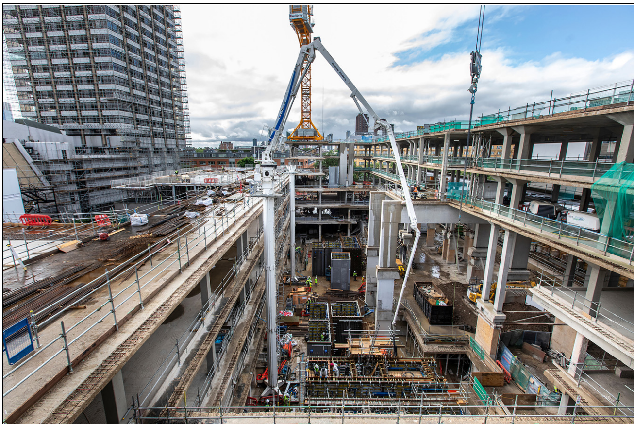
Figure 11. Demolition and construction
