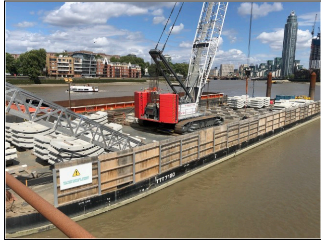
Figure 5. Main tunnel segment delivery by barge
