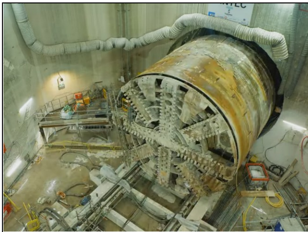
Figure 10. TBM C transitioning from reception chamber to cradle
