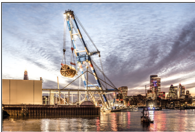
Figure 11. A 1800 t sheerleg crane lifts TBM C, named Ursula, after cryobiologist Dr Audrey Ursula Smith (© tobyhawkes.co.nz)
