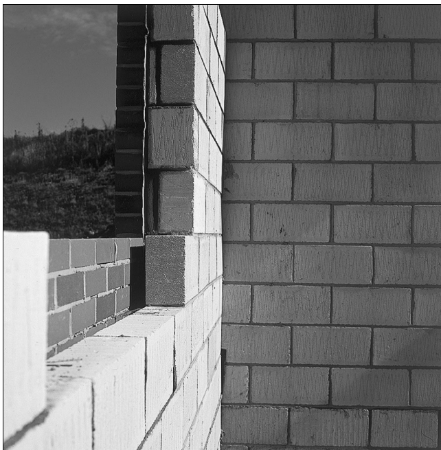
Fig. 4. Inner leaf construction in external wall (courtesy of H + H Celcon Ltd)
