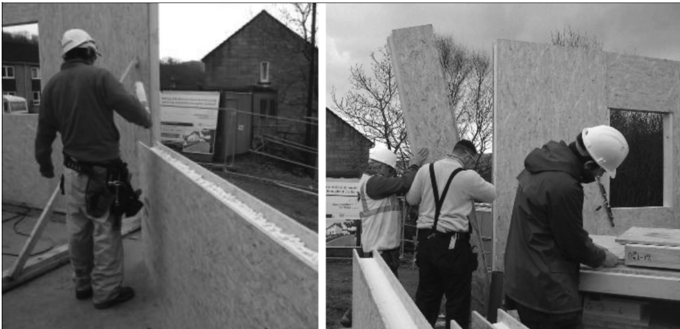
Fig. 1. Structural insulated wall panels during construction
