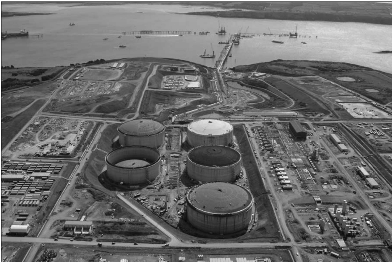
Fig. 1. South Hook liquefied natural gas storage tanks
