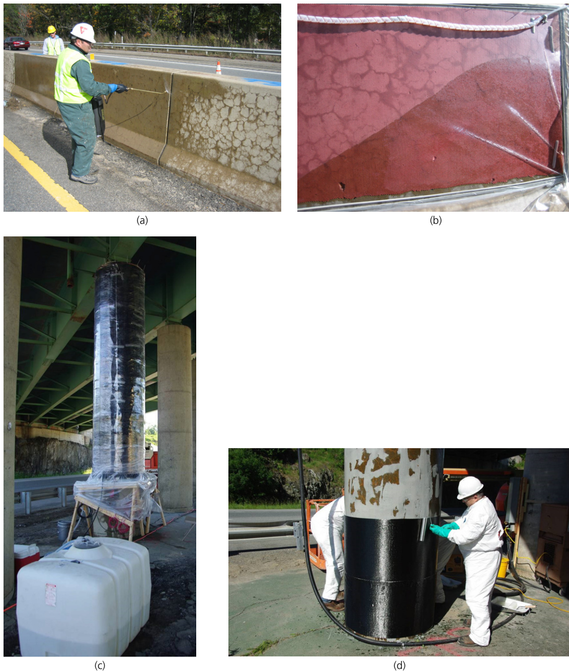
Figure 2. Mitigation methods/materials: (a) topical application of lithium nitrate, (b) vacuum application of lithium nitrate, (c) electrochemical application of lithium compounds and (d) FRP wrap of column
