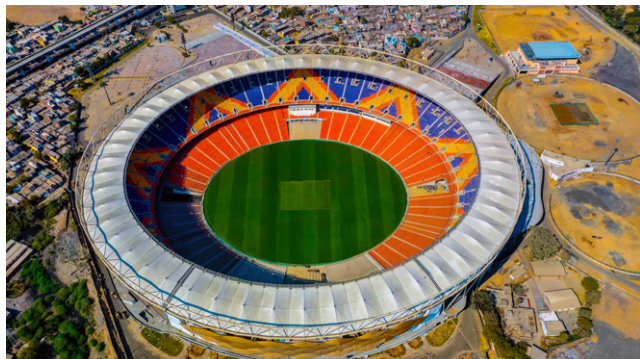
Figure 1. Bird's-eye view of Motera Cricket Stadium
