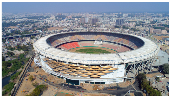
Figure 2. Motera Cricket Stadium
