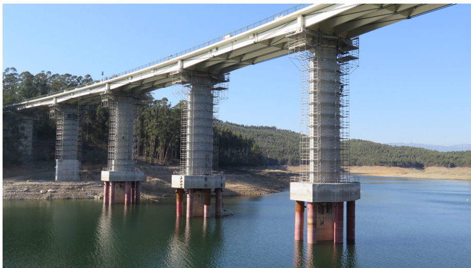
Figure 1. Criz II Bridge at the end of the rehabilitation works (Santos et al. , 2022)
