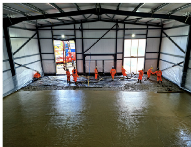
Figure 1. Solstice Park development: slab pour with graphene infused concrete underway
