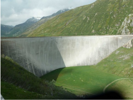
Figure 10. Nalps dam – downstream face
