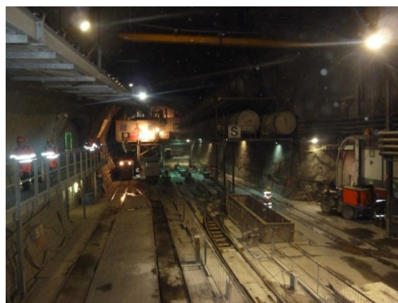
Figure 4. Underground railway tunnel
