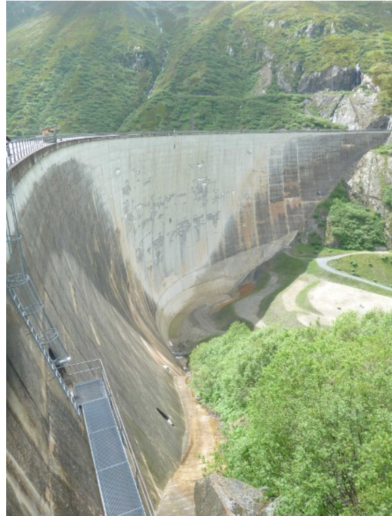
Figure 8. Nalps dam downstream – fill removed at toe
