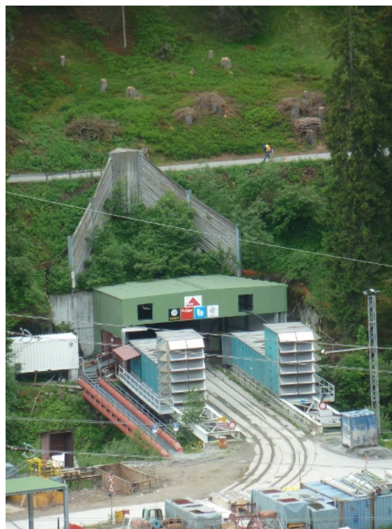
Figure 3. Entrance to tunnel works
