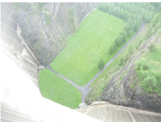
Figure 12. Luzzone arch dam – gated spillway
