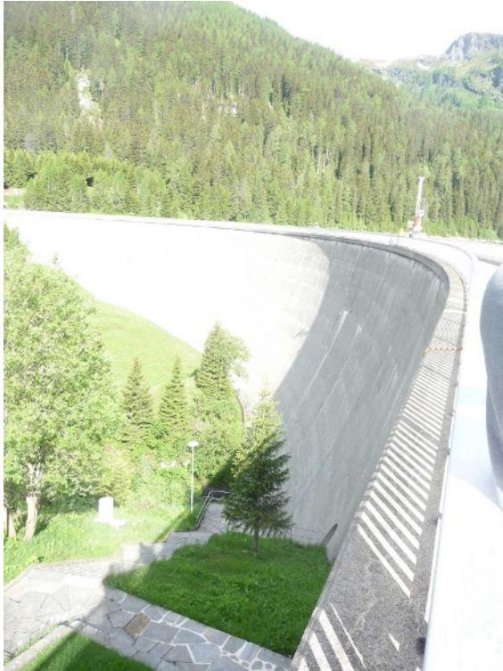
Figure 16. Isola dam – downstream face
