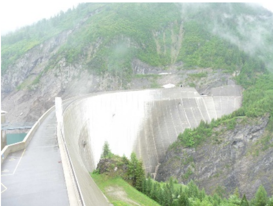
Figure 11. Luzzone arch dam – downstream face from crest
