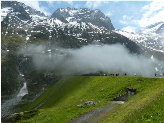
Figure 3. The grassed downstream slope of Göscheneralp dam
