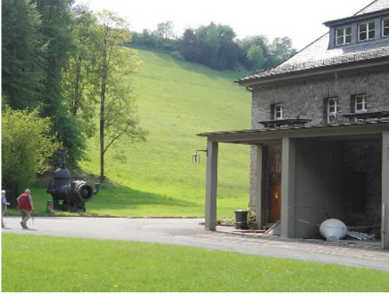
Figure 1. Downstream face of Sorpe dam
