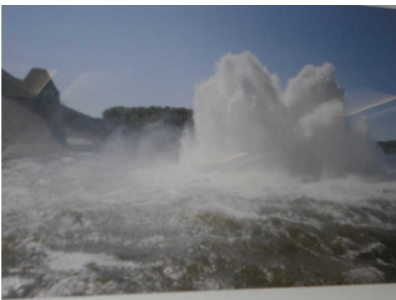
Figure 3. Flow from the bottom outlet is shot vertically into the air downstream of the dam
