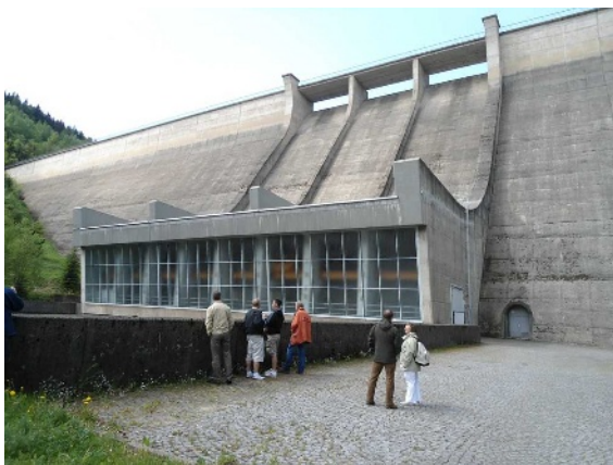
Figure 7. Eibenstock dam with spillway and valve house
