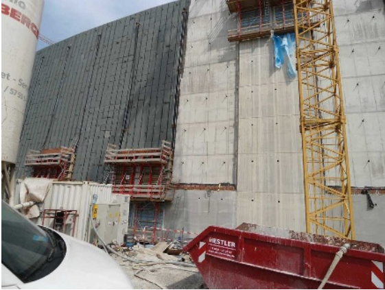
Figure 12. Application of impermeable facing to Klingenberg dam
