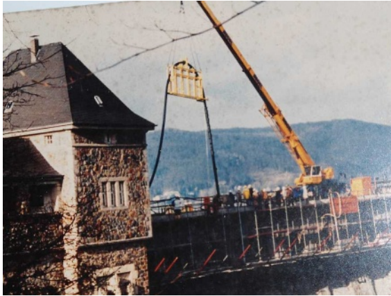
Figure 6. Old photograph showing installation of anchors in 1991–1994
