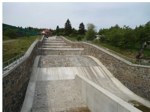
Figure 11. Restored spillway at Klingenberg
