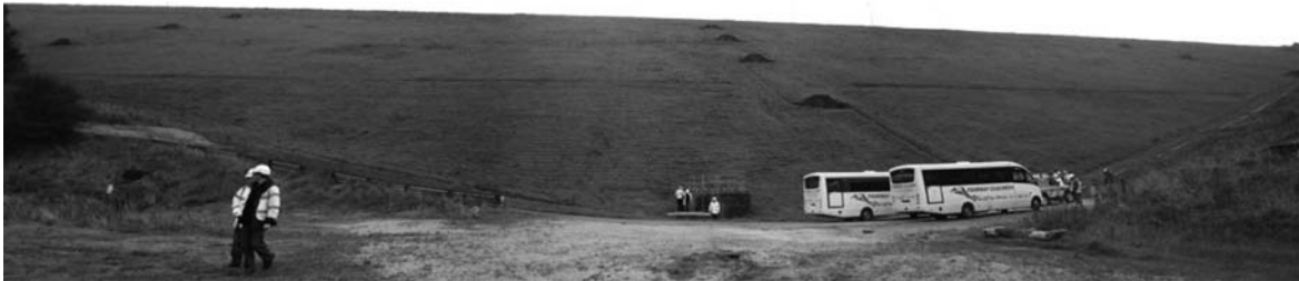
Figure 3. Scammonden embankment panorama with tour members and coaches
