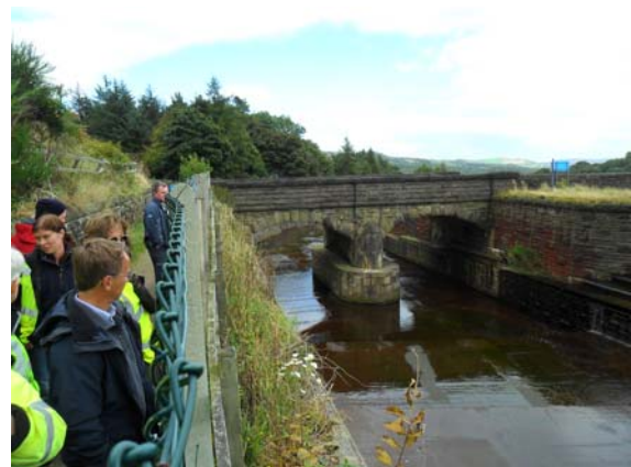
Figure 2. Delegates viewing the lowered spillway channel at Langsett reservoir
