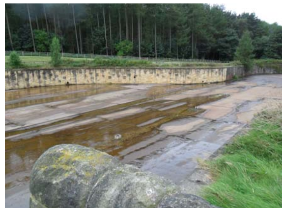
Figure 3. Widened upper section of spillway channel at Underbank reservoir
