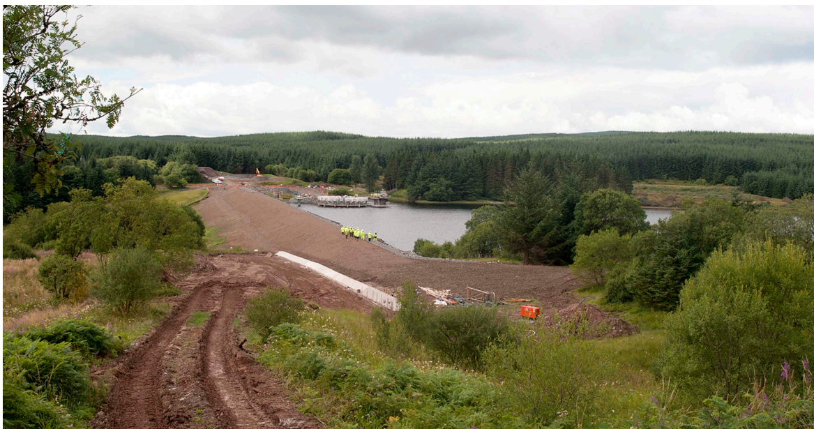
Figure 2. General view of site during tour, with one tour group on the dam crest and the other on the bellmouth and valve tower at the far side
