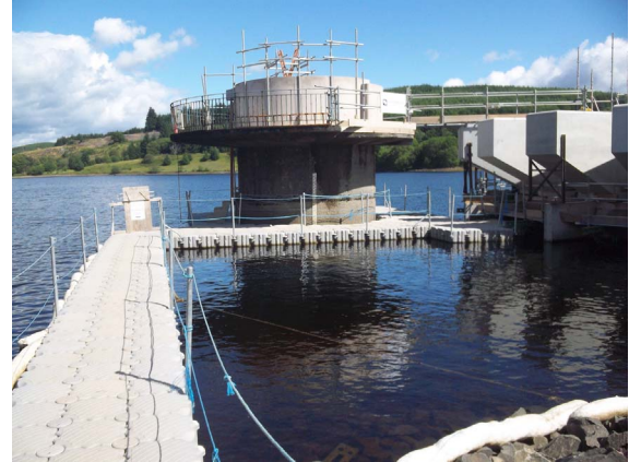
Figure 3. Floating pontoon access platform at valve tower and bellmouth spillway
