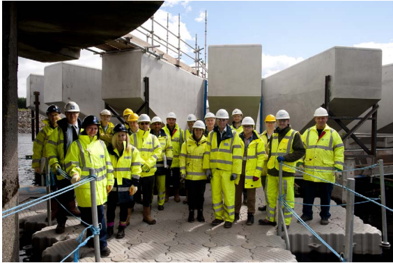
Figure 4. One of the two tour groups up close with the new piano-key spillway
