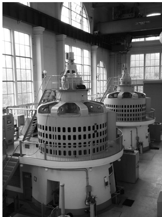
Figure 4. Cushman dam no. 2 power house turbines
