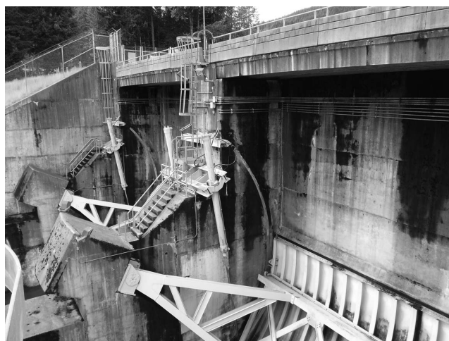
Figure 7. Cushman dam no. 1 spillway radial gates
