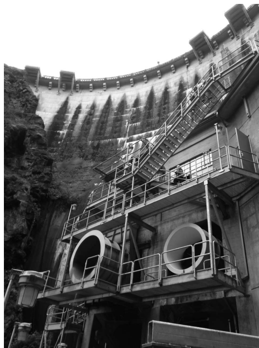
Figure 1. Cushman dam no. 1
