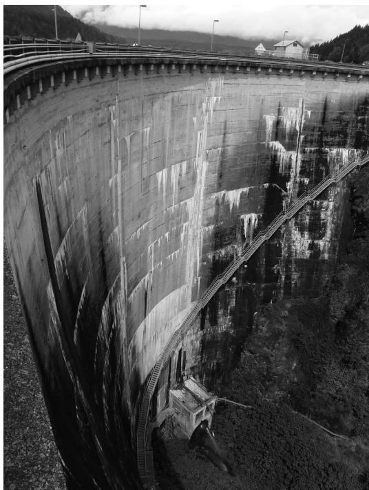
Figure 2. Cushman dam no. 2
