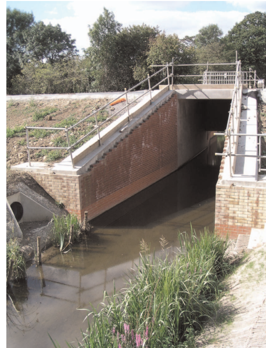
Figure 3. Flume with cantilevered sheet pile walls
